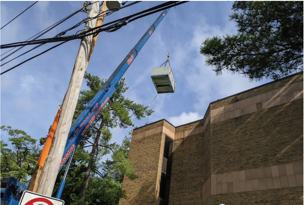
The old sanctuary air conditioning and heating units were removed from the roof and replaced with a new powerful system.
